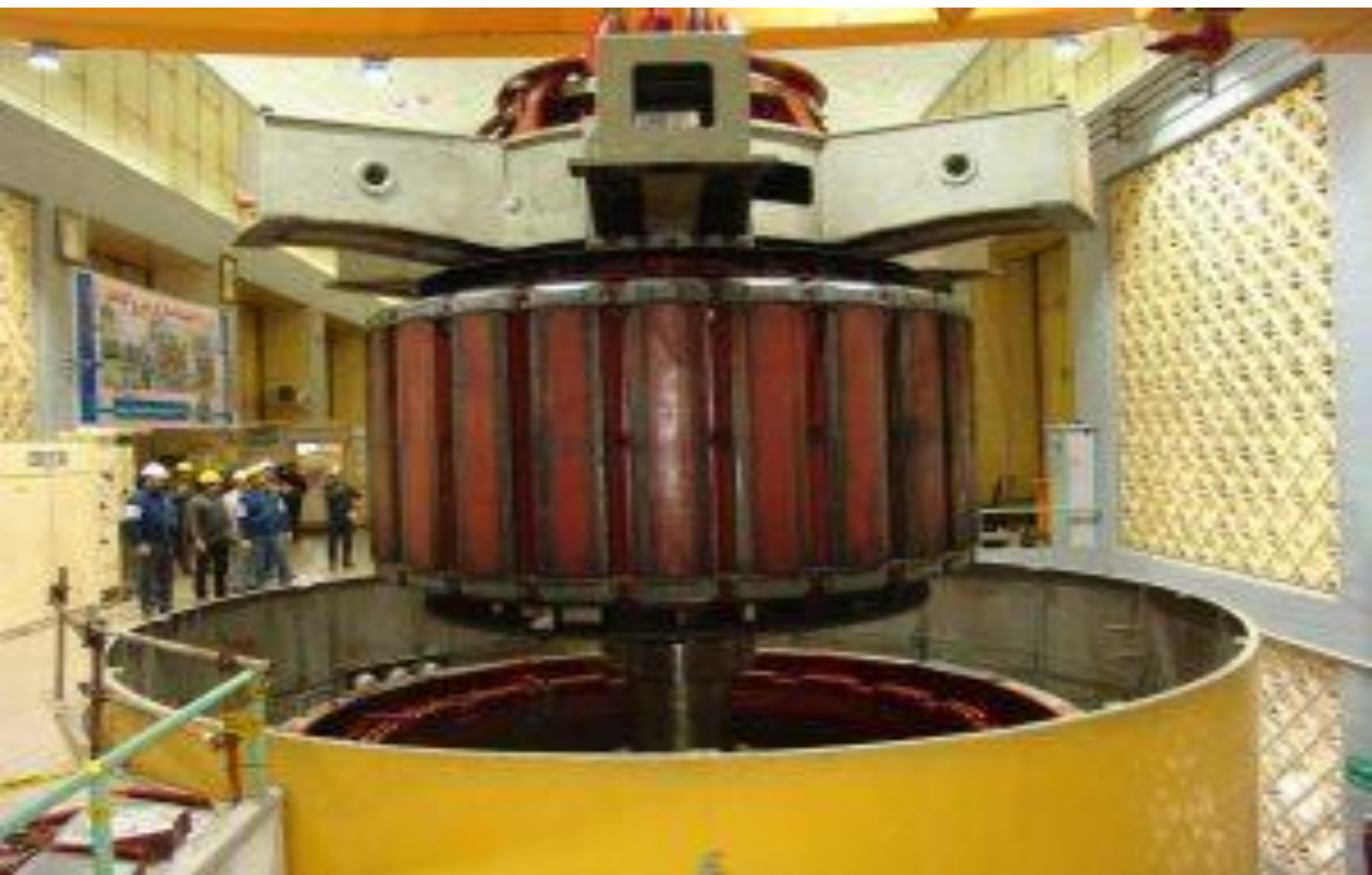
Rotor and stator of a 90 MW, 22-pole hydro generator at the Dez Power Plant, Dezfool, Iran.
