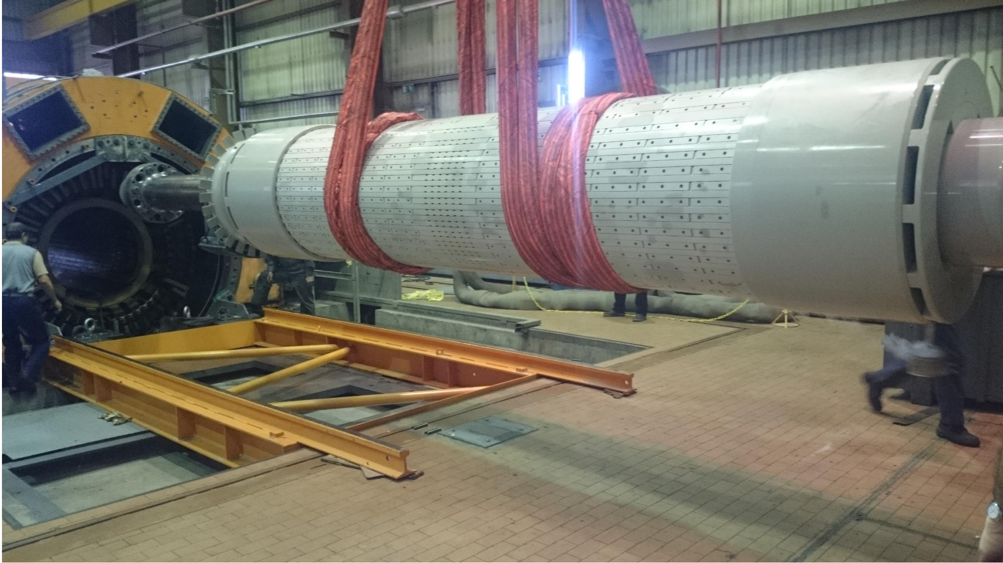
Rotor and stator of a 160 MW, 2-pole generator at the Toos Power Plant, Mashhad, Iran.
