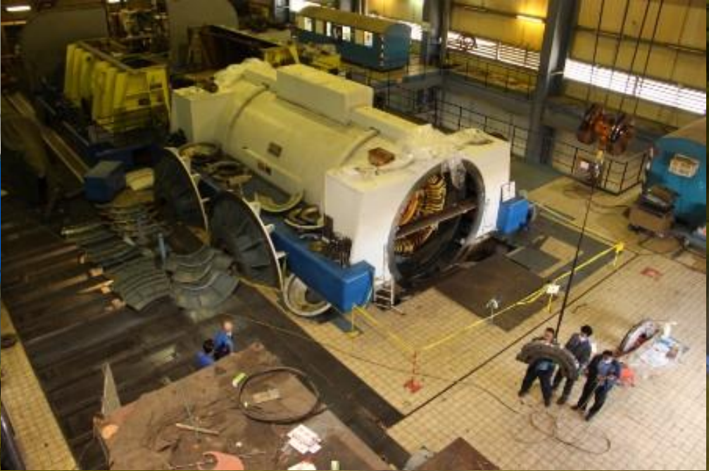
Rotor and stator of a 440 MW, 2-pole turbo generator at the Shahid Salimi Power Plant, Neka, Iran.
