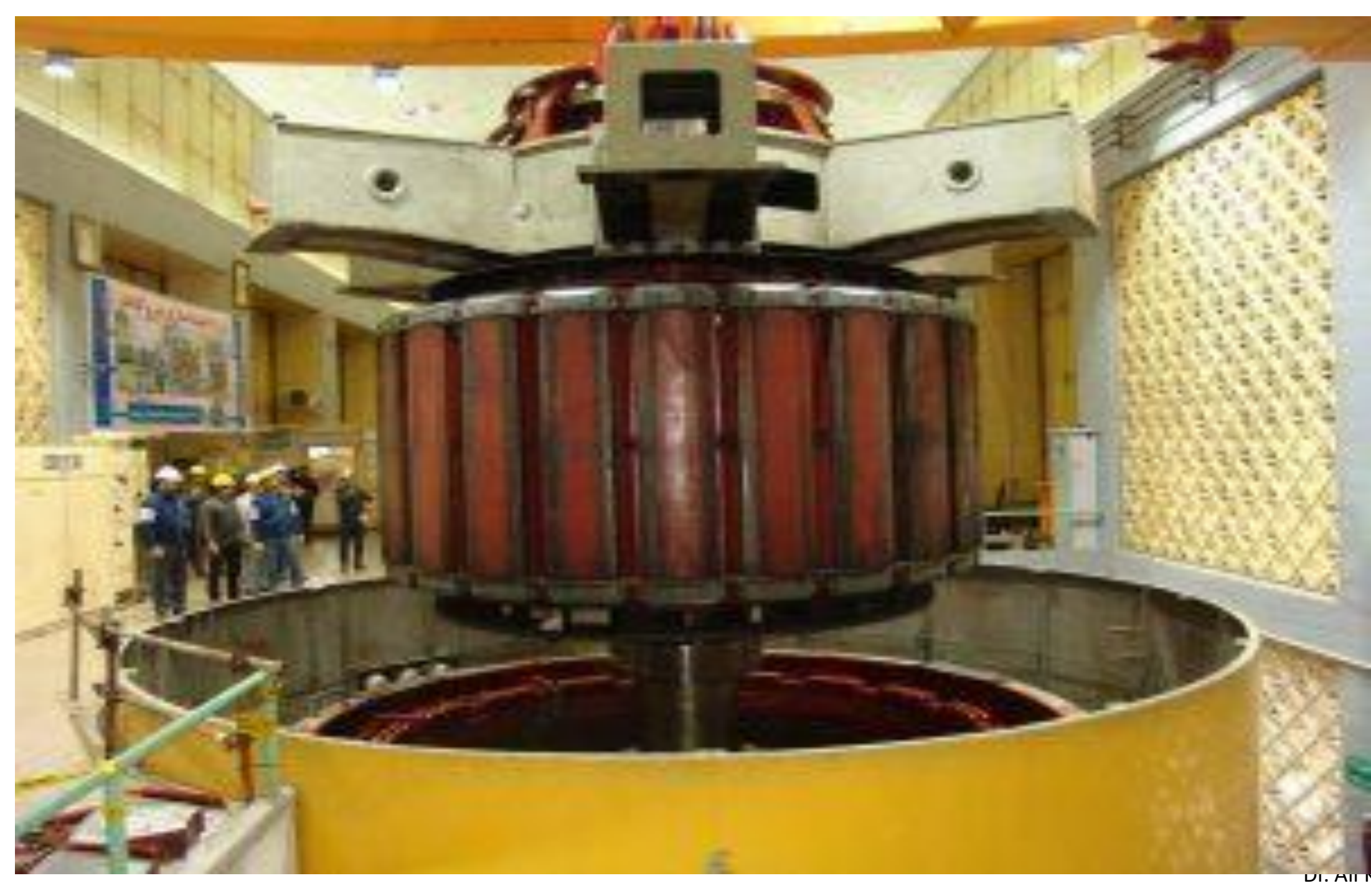
Rotor and stator of a 90 MW, 22-pole hydro generator at the Dez Power Plant, Dezfool, Iran.
